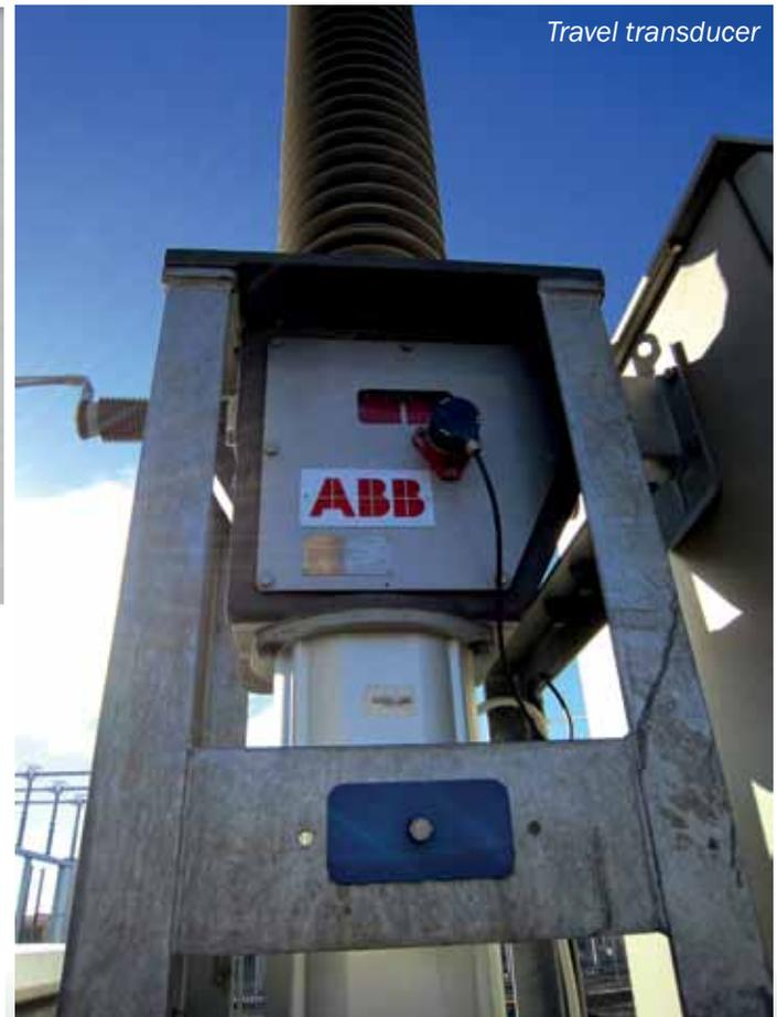
**OLM2 continuously monitors circuit breaker condition. It signals in real time any malfunction to maintenance services. Therefore, OLM2 facilitates reduced maintenance cost and failure risk.**
